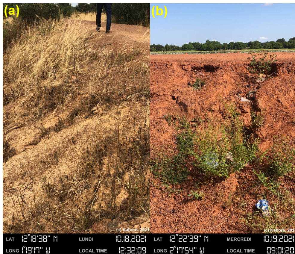
Figure 4. (a) Gully on a downstream slope, Petit Tansobentenga dam (Centre Region). (b) Gully on a downstream slope, Godin-Oudalogtinga dam (Centre-West Region).
